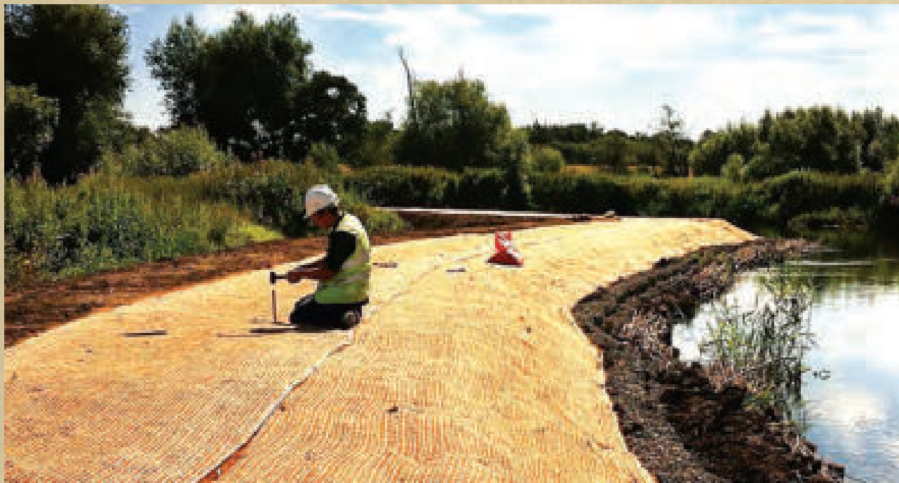
Geotext tiles in protection of river banks
