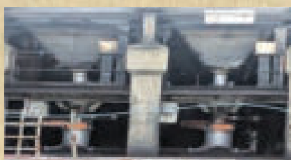
ESP Boiler Fly Ash collection system
