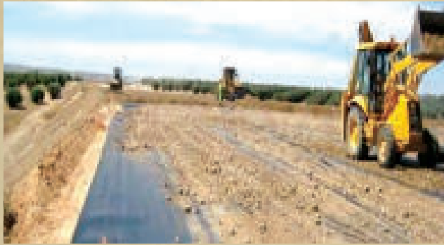
Geo-textiles in road construction
