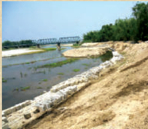
Geo-textiles in slope stabilization
