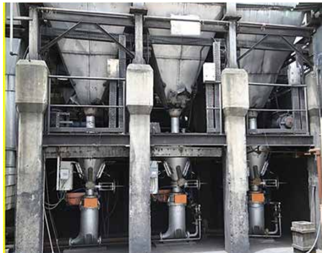
Activated carbon chambers for the Effluent Treatment Plant
