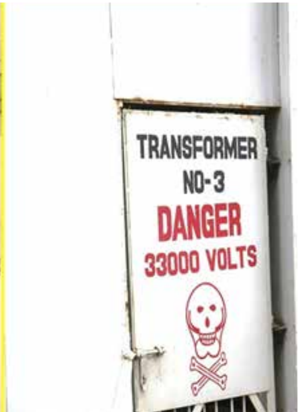
33 KV transformers installed in place of 6 KV Transformer to receive GRID Power to Reduce losses
