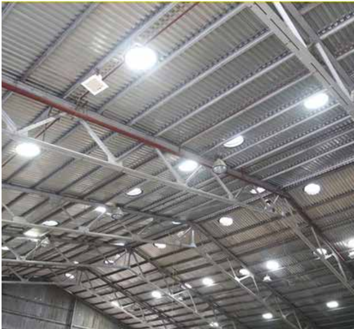
Solar Lighting system used in our Process areas
