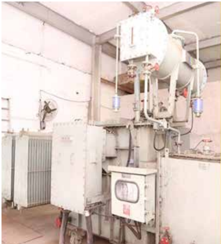
33 KV transformers installed in place of 6 KV Transformer to receive GRID Power to Reduce losses
