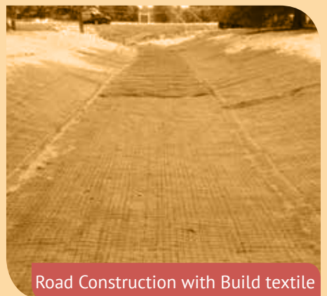
Slope stabilization with Geotextile
