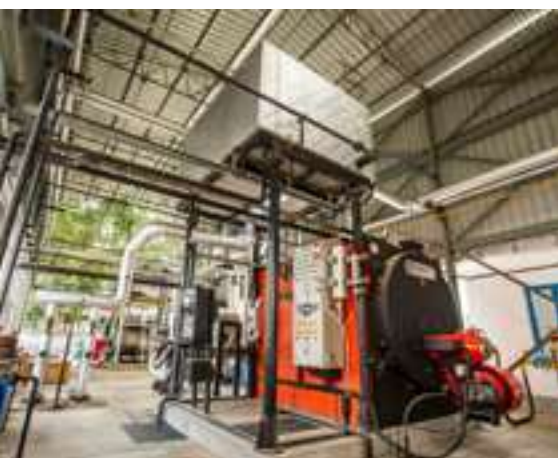
New gas fired boiler at Ananya plant
